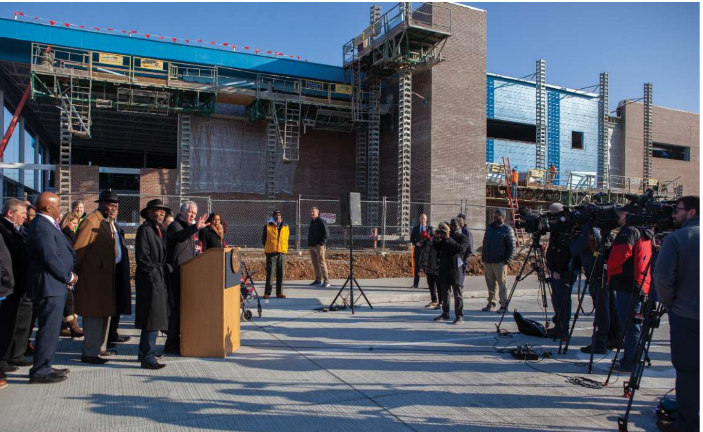
Community leaders discuss the construction progress of West Louisville's new Republic Bank Foundation YMCA.
